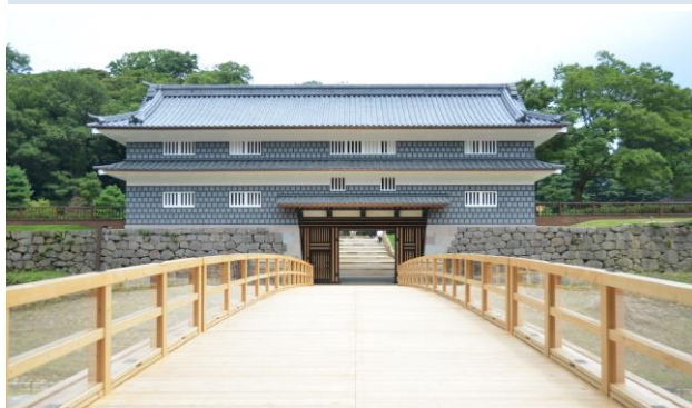
“金沢城鼠多門・鼠多門橋” “Kanazawa castle Nezumitamon Gate and Bridge”
